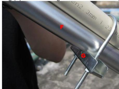
9. Hoist Mast up and make sure plumb at 90° angle. Ensure antenna is at least 3 feet from ground and above all surrounding obstructions such as roof tops, trees, hills, walls, etc.
